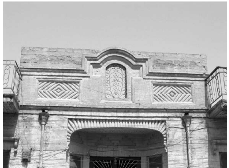
Figure 1.8. Sculpted detail in brick, Battaween, east bank. Most façades mix Art Deco stylization and revisited traditional forms, circa late 1920s. The gutters of cast-iron and wrought-iron balcony fence were imported from England. (Pieri 2008: 133)
