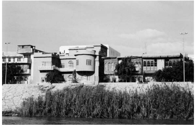
Figure 1.6. Baghdad, Sinak, east bank. Continuity between the transitional houses of the late 1920s, of brick and wood, and the houses of the 1940s, brick coated with cement. (Pieri 2008: 72)
